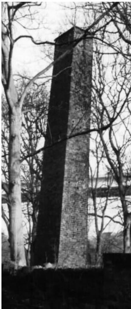
Chimney to the east of site, viewed from the rear
