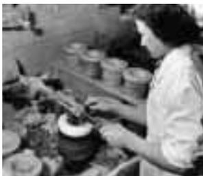
This department was the most difficult and strenuous in which to work and wages were paid (as in all the making departments) only on what the Jolleymen could produce. On average, about two thousand articles were made by each machine in an eight hour period. The cups and holloware were then taken to the Topping and Turning shop where they were shaped, turned and polished by the use of hand tools.
